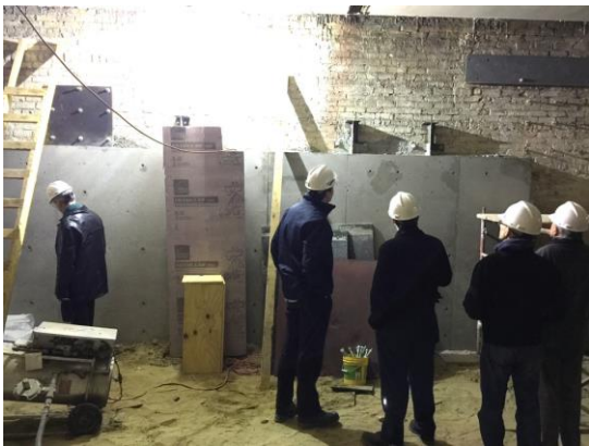
Fig. 2. Inspecting recently-unveiled basement walls.
