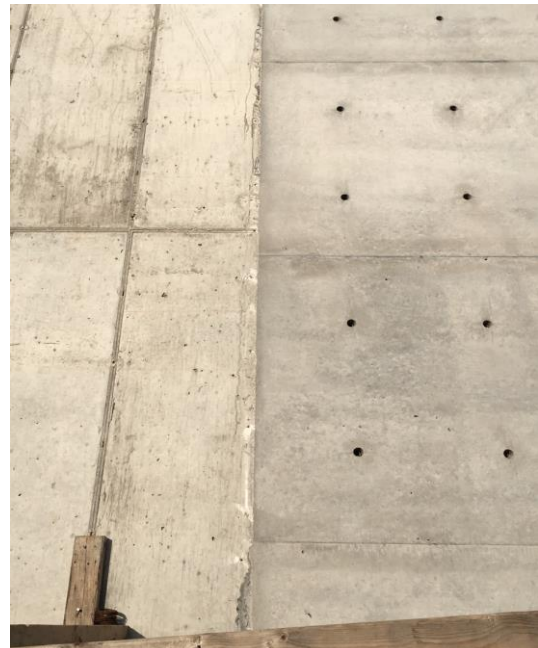
Fig. 6. Left: Symons gang form impression; Right: FinnForm face.
