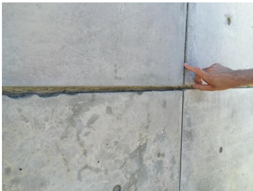
Fig. 10. Post-stripping of mock-up number 1; detail.
