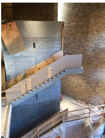
Fig. 15. Staircase cantilevered from 'fin' wall.
