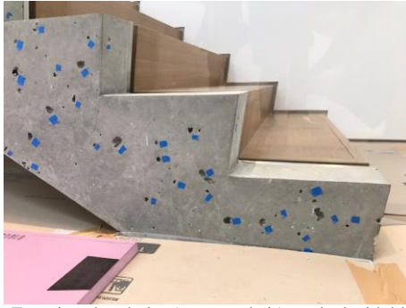
Fig. 12. Egregious bug holes (entrapped air) marked with blue tape.
