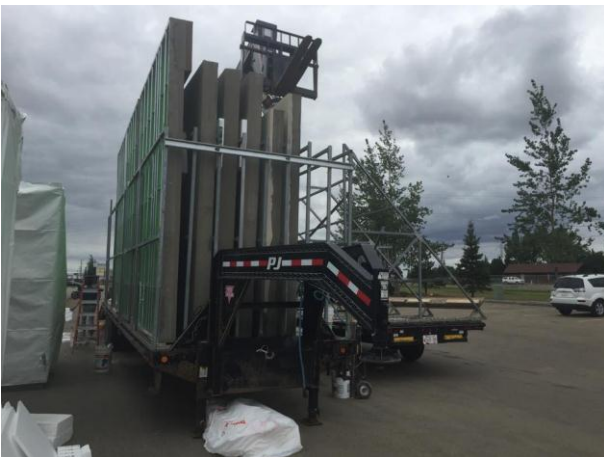
Fig. 8. Alignment of panels on trailer.
