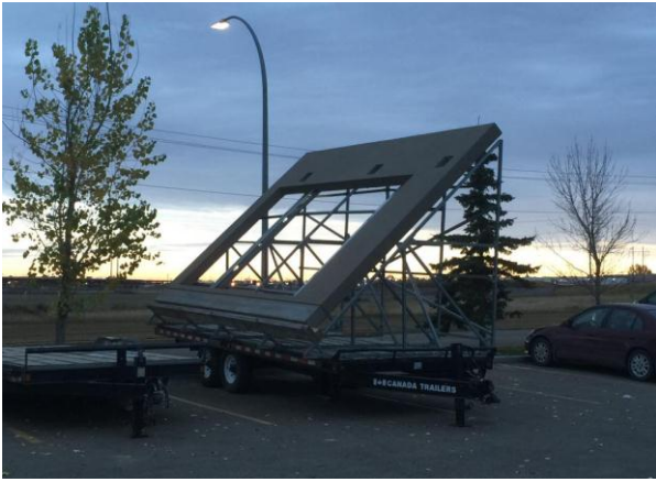
Fig. 10. inclined steel frame for last floor parapet panel transportation.
