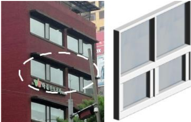
Fig. 3. Examples of windows in existing buildings.
