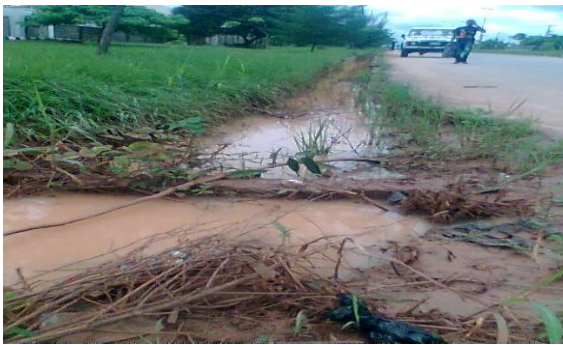
Fig. 2. Water log in a concrete drain.
