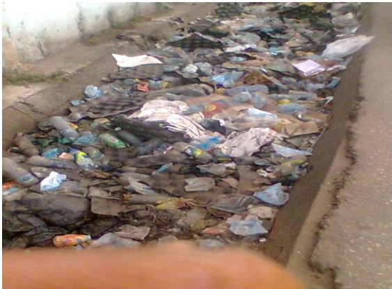
Fig. 1. Waste dump in a concrete drain.
